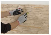
Let the putty dry for approximately 24 hours (this time will depend on the room temperature) and touch up the joints and holes where the putty has been applied with Panespol touch-up paint.
