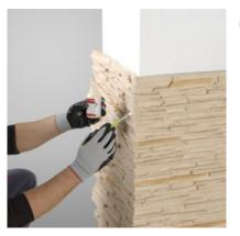
Let the putty dry for approximately 24 hours (this time will depend on the room temperature) and touch up the stones and bricks, where necessary, with Panespol touch-up paint. Once this paint is dry, finish the joints area with Panespol touch-up paint for the joints.
