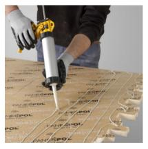
Once each part of the panel has been cut at 45°, apply the adhesive on the back of the panel creating a bead. Attention: consult in case of outdoor installation as a specific adhesive will be used.
