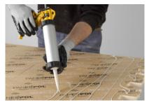
Apply the adhesive on the back of the panel creating a bead. Attention: consult in case of outdoor installation as a specific adhesive will be used.
