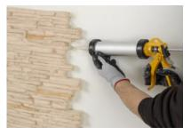
Once the first panel is fixed, apply a bead of adhesive on the perimeter of it.
