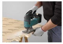
With a jigsaw cut the ends of the panel to begin the assembly at one end of the wall.
