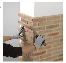
Screw together the two pieces that cover the corner with 2 or 3 screws (depending on the height). Spread the adhesive with the help of a brush shaping it to the panel. Then screw the second piece of the corner to the wall. If necessary, file the irregularities of the angle.
