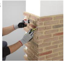
Finally, with the help of a fine brush or cloth, touch up the panels with the pigment applied dry until the desired result is obtained.
