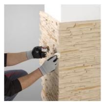
Finally, with the help of a fine brush or cloth, touch up the panels with the pigment applied dry until the desired result is obtained.
