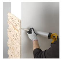
Once the first piece of the corner is placed, apply a bead of adhesive to the mitre and place the other piece. The joint needs to be tight together so that it presses the adhesive.
