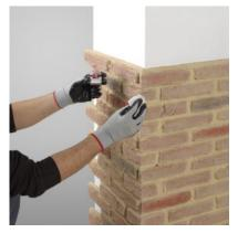
Let the putty dry for approximately 24 hours (this time will depend on the room temperature) and touch up the stones and bricks, where necessary, with Panespol touch-up paint. Once this paint is dry, finish the joints area with Panespol touch-up paint or the joints.
