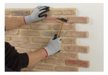
Prepare screws inside plugs previously and introduce them into the holes made in the panel and wall with the help of a hammer. Next, screw until the screw is inserted without going through the panel. We recommend screwing the entire perimeter and the central part. (Use about a dozen screws per m2, double for outdoor applications.)
