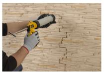
Cover with putty the holes of the screws and the joint between the panels.
