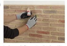
Let the putty dry for approximately 24 hours (this time will depend on the room temperature) and touch up the joints and holes where the putty has been applied with Panespol joint paint.
