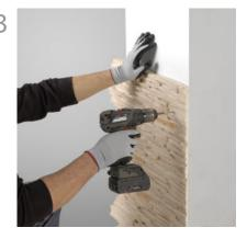
Place the panel on the wall and drill panel and wall simultaneously. Prepare screws inside plugs previously and introduce them into the holes made in the panel and wall with the help of a hammer. Next, screw until the screw is inserted without going through the panel.
