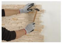
Prepare screws inside plugs previously and introduce them into the holes made in the panel and wall with the help of a hammer. Next, screw until the screw is inserted without going through the panel. We recommend screwing the entire perimeter and the entral part. (Use about a dozen screws per m2, double for outdoor applications.)
