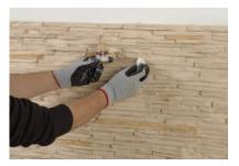
Finally, with the help of a fine brush or cloth, touch up the panels with dry-applied pigment powder until the desired result is obtained.
