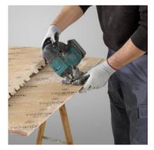
Place the panel on the corner and draw a line on the back of the panel that will be used to make the miter cut. Cut the panel at 45° with a jigsaw following the line previously marked.
