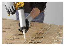
Apply the adhesive on the back of the panel creating a bead. Attention: consult in case of outdoor installation as a specific adhesive will be
