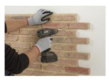
Drill panel and wall simultaneously. Make these holes in the areas of the joints, since later the retouching will be easier to carry out.
