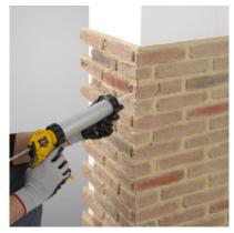
Once all the panels are assembled, cover with putty the holes of the screws and the joint between the panels.
