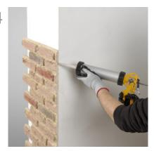
Once the first piece of the corner is placed, apply a bead of adhesive to the mitre and place the other piece. The joint needs to be tight together so that it presses the adhesive.
