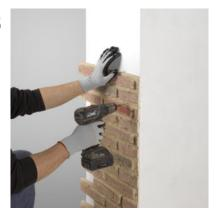
Place the panel on the wall and drill panel and wall simultaneously. Make these holes in the areas of the joints, since the retouching will be easier to carry out. Prepare screws inside plugs previously and introduce them into the holes made in the panel and wall with the help of a hammer. Next, screw until the screw is inserted without going through the panel.
