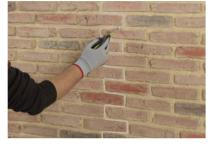
Spread the putty with the help of a brush giving it the appropriate shape all along the joint.
