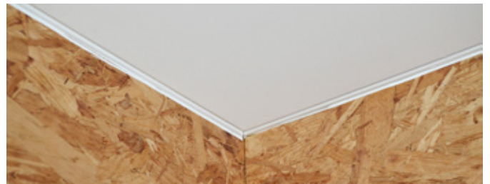
Image B05 - corner assembly – with textile
