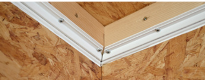
Image B04 - corner assembly – shell
