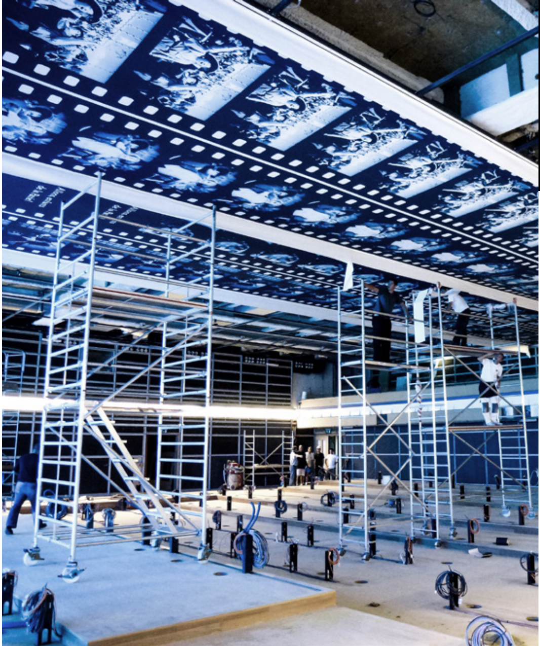
Image B58 - Hôtel de Ville de Montpellier (Montpellier, France) Architects: Jean Nouvel (Ateliers Jean Nouvel), Francois Fontès (Francois Fontès Architecture) Implemented solution: Digitally printed DESCOR® PREMIUM Acoustic
