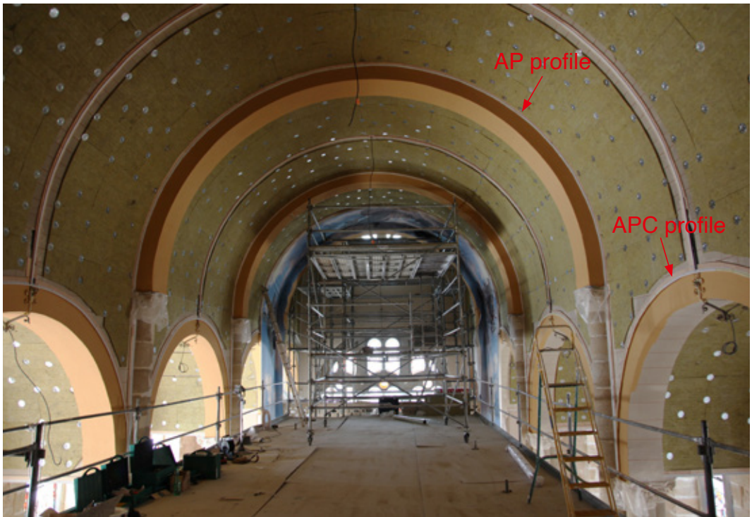
Image B16-B18 - AP profile, APC profile and insulating material in application
