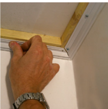
Image B06 - corner assembly – shell
