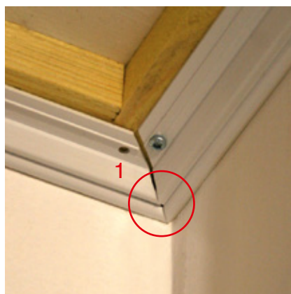
Image B06 - corner assembly – shell
